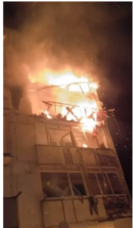
Source: Press Service of the Zaporozhye Region Governor. Date: March 8, 2026.
